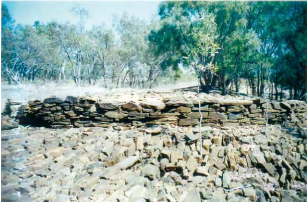
Figure 6 Stone pitched spillway and abutment.
