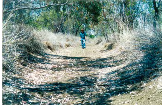
Figure 7 Channel excavated to feed off-stream storage dam.
